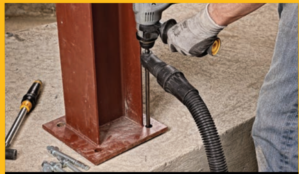
➤ Dust X+™ anchor installation system
